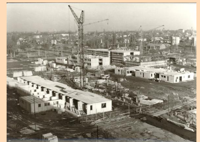
Havanna housing estate in construction
